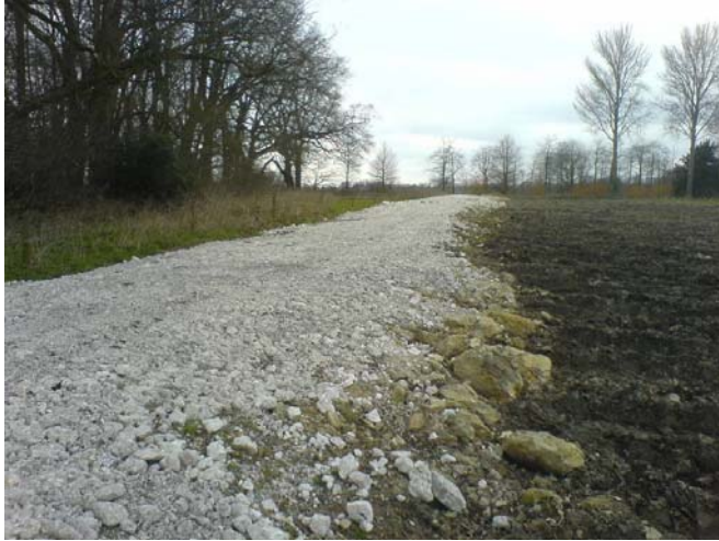
Crown almost flat for comfortable cow walking
