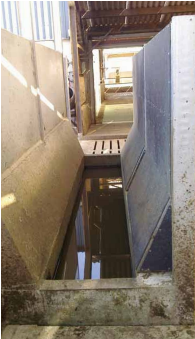
Figure 1. Long, narrow and high-walled foot bath design has been advocated by some authors as this increases foot immersion time (Cook et al 2013) and reduces kick-out losses of footbath solution.
