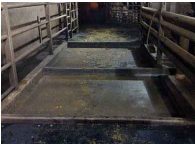
Figure 2. Wide footbaths (>1.8m) that allow cows to pass are considered optimal for cow flow in positions close to the parlour (Chesterton 2013). Some authors suggest the pre-rinse footbath is unnecessary (Cook et al 2012) although no reports have directly measured levels of contamination with or without the pre-rinse.
